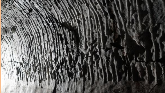
Photo 24. Regular vertical fluting on wall.
